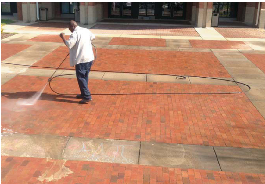
A brick paver surface that's acceptable for street painting.
